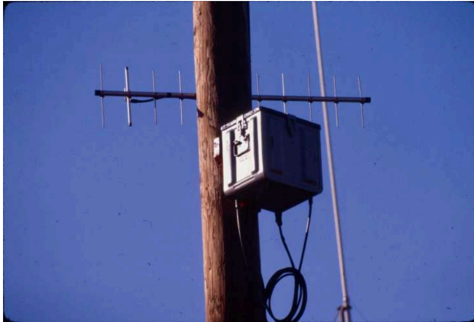
The Maugus Hill remote receiver and UHF link in 1981.
